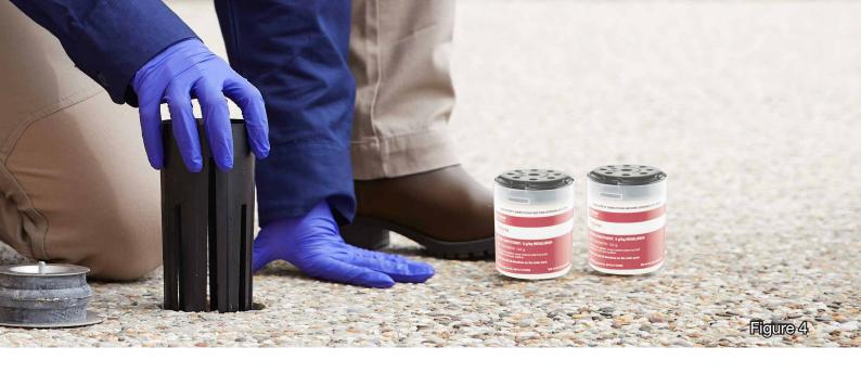
To create the required opening for the ATBS inground station, an auger of 75-80mm is required and a hole should be excavated to a depth of at least 170mm to allow the station to be installed to a neat finish, close to the ground level. If possible, it is recommended that the hole is excavated an additional 50-80mm below the depth of the base of the station to create a natural sump to allow the excess moisture to drain (Figure 1).
